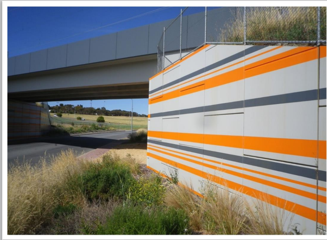
Seaford Rail Corridor
