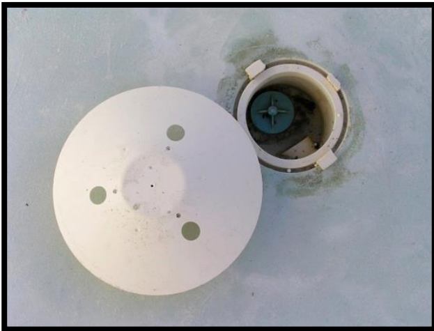
Fig 1: Typical hydrostatic valve assembly
