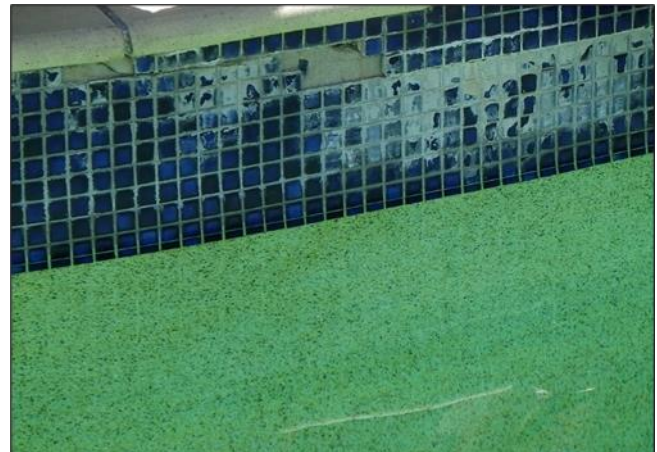
Figure 2 So many water related issues resulting in tiles being lost. Note the area below the tiles, being porous it looks OK.
