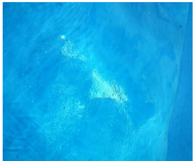
Figure 2. Not enough uniform spreading out, so worn off too soon in some areas.
